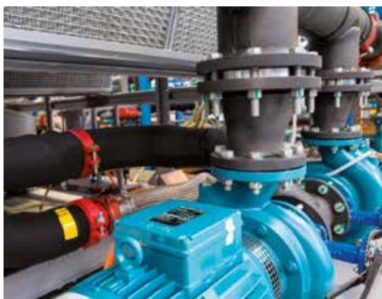
Choosing the best solution for pumps is certainly one of the most important challenges for the designer. Uniflair Chillers have an onboard pump group which can be inverter-driven.
